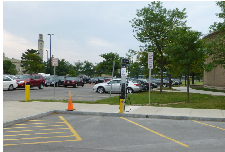
Level 2 charging station at Diefendorf Hall on University of Buffalo's South Campus. Photo credit: Energetics
