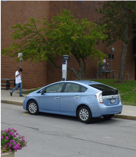
Level 2 charging station at Bonner Hall on University at Buffalo's North Campus. Photo credit: Energetics
