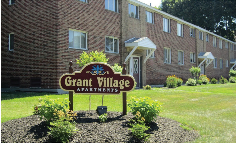
Grant Village Apartments, Syracuse, NY. Photo credit: NYSERDA
